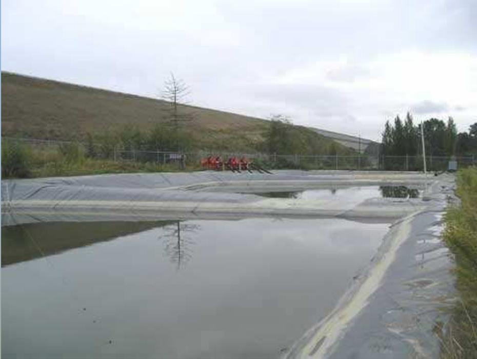
Port of Seattle stormwater detention pond with SeaTac Airport third runway in the distance. After being treated, stormwater is discharged to Miller Creek.
