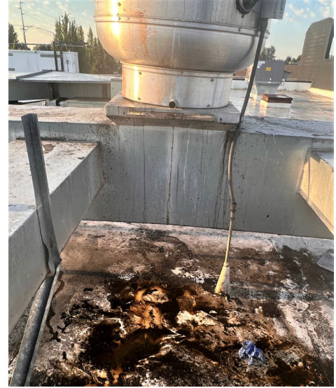
Grease buildup on rooftop can overflow into your roof drain and onto your parking lot, where the pollution is carried to local waterways.
