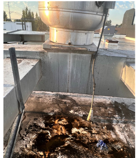
Grease buildup on rooftop can overflow into your roof drain and onto your parking lot, where the pollution is carried to local waterways.
