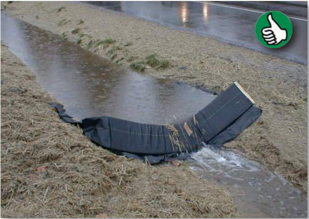
Good example of a properly installed check dam. (Source: WSDOT)
