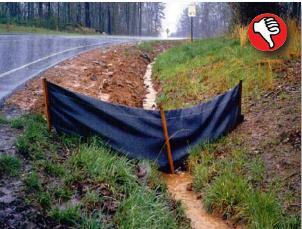
Silt fence is not an approved BMP for use as a check dam. (Source: Peter Vaughn, A3E Consultants)
