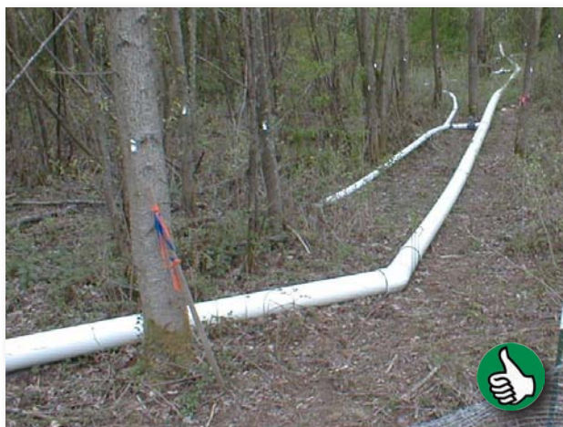
Six inch pipe draining a sediment pond. The six inch pipe drains into four inch perforated pipe which allow the sediment laden water to percolate through the duff and soil. (Source: WSDOT)
