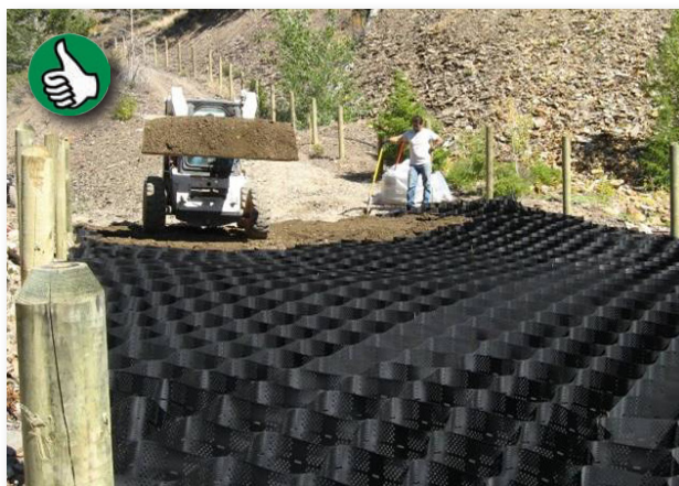
Example installation of cellular confinement system. (Source: TerraGraphics Environmental Engineering, Inc., via Peter Vaughn, A3E Consultants)
