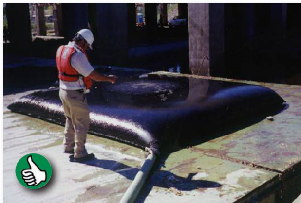
Sediment bag used to clean sediment laden water. (Source: WSDOT)
