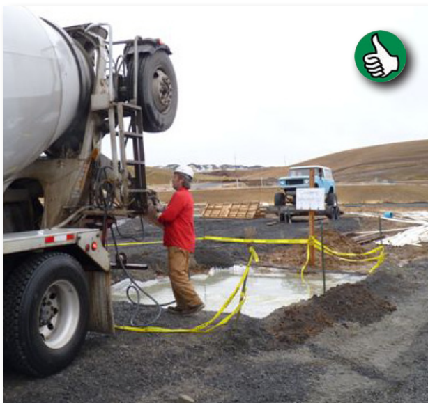
Good example of properly designed concrete washout area. (Source: City of Pullman)
