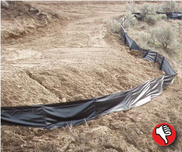
Silt fence is installed backwards; posts should be on downhill side. (Source: City of Wenatchee)
