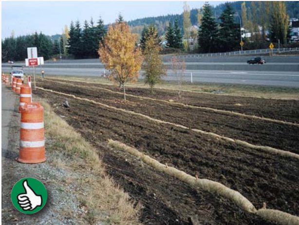
Good example of properly installed wattles.
