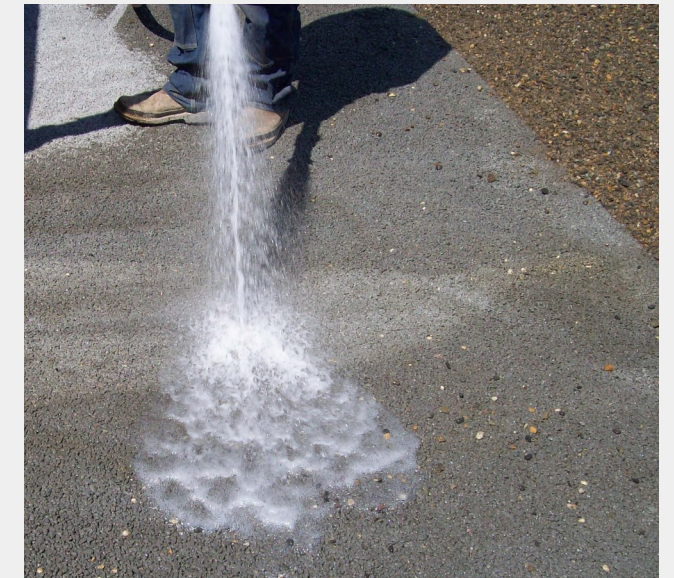
Runoff infiltrates through permeable pavement.
