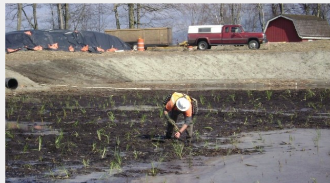
Constructed stormwater wetland during construction.
