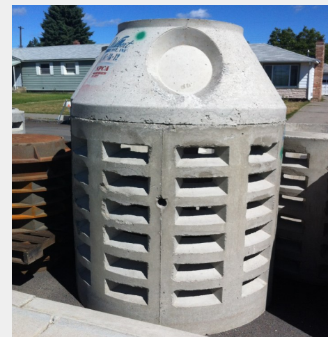
Drywells are an example of a UIC.
