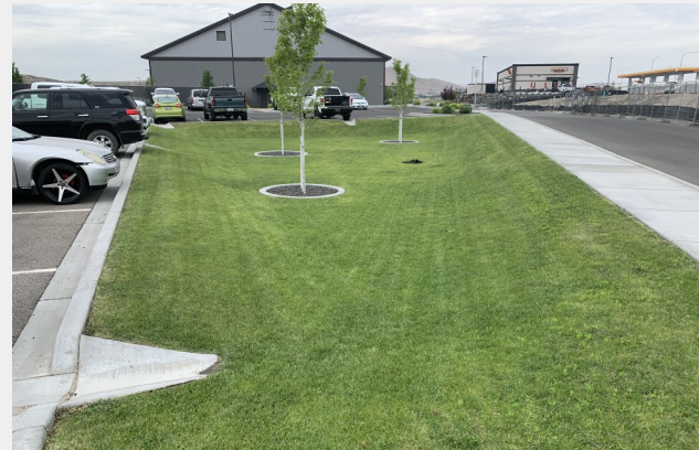
Bioinfiltration BMP in Eastern Washington.
