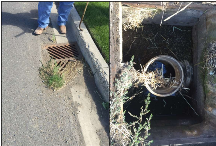
Figure 3.3 Proposed study area: typical roadway and catch basin sediment accumulation
