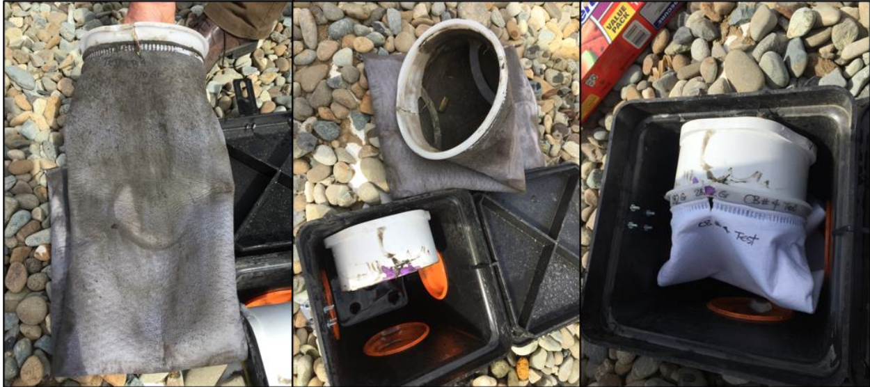
Figure 5.7 Catch Basin Socks: after 2 months use (left), uninstalled (middle), installed and new (right)
