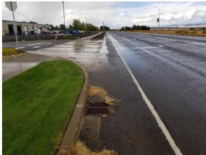
Figure 3.9 Approaches contribute runoff to catch basins
