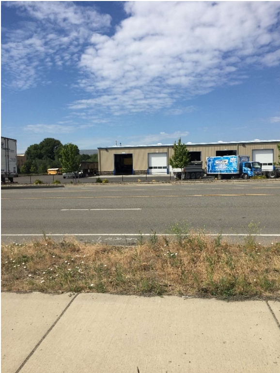
Photo of a closed sump box at the site and the upstream/area across the street
