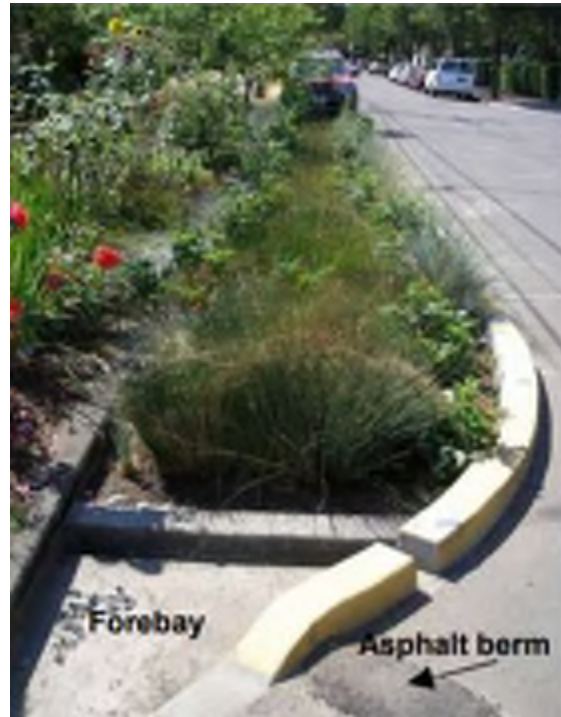
Figure 2: Curb Extension with Concrete Forebay
