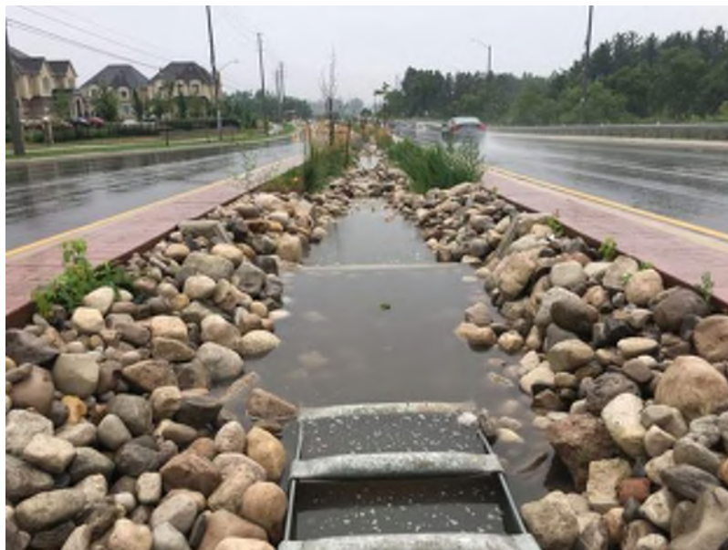
Figure 3: Rock-Lined Forebay in Swale
