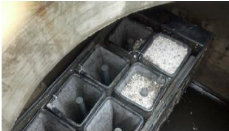
Installation of temporary perlite prefilter with new cartridge design
