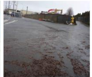
High sediment loading in drainage basin
