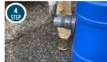
4 STEP Install 4-inch schedule 80 PVC threaded nipple on to bulkhead fitting.
