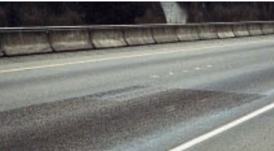
Chip Seal Repair Low
