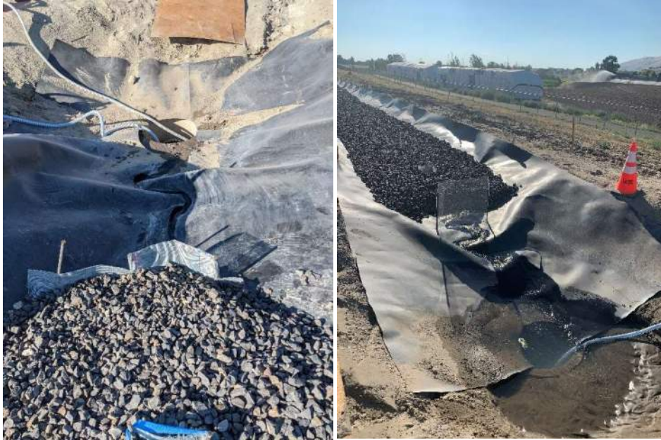
Figure 4-6. Facing downgrade from end of swale to catch basin
