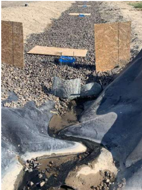
Figure 4-7. Weir installed following Event 4, facing upstream
